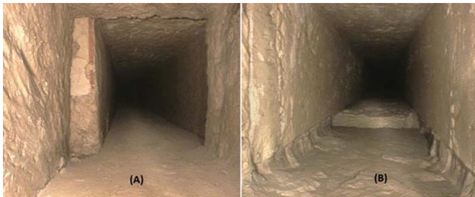
Figure 3. Major obstacles within the southern shaft: (A) lateral displacement, (B) floor step (Gantenbrink, 1999).
